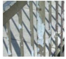
Some manufacturers galvanise their fencing for a longer life, but paint straight on top of it – again poor appearance and high maintenance
