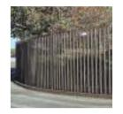
from low to high security. Through visibility is poor and will not work effectively with CCTV cameras. The draconian appearance may not be acceptable to the local community.
