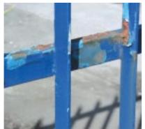
Metal fencing without a galvanised finish is prone to rusting – resulting in poor appearance and high maintenance costs
