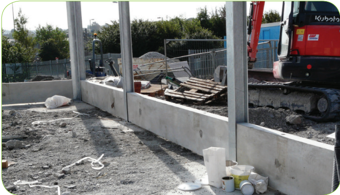
● Concrete Plinth to establish level.
