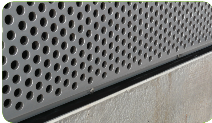
● Base gasket secured to concrete plinth.
